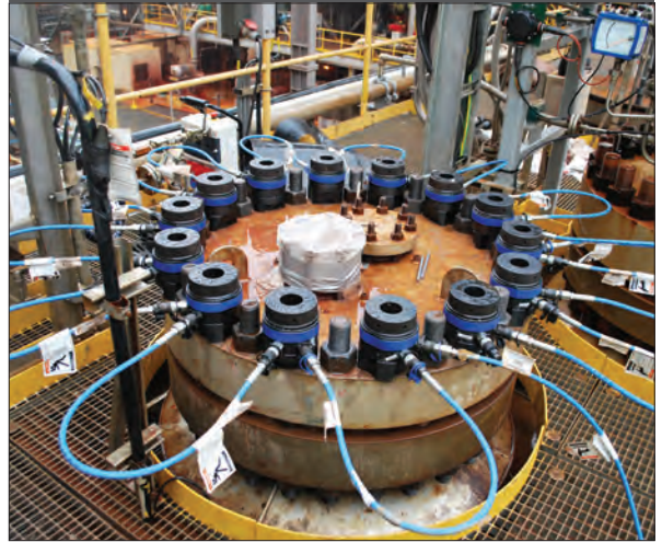
▲ Custom tensioners used for tensioning multiple bolts on pipe line flange
