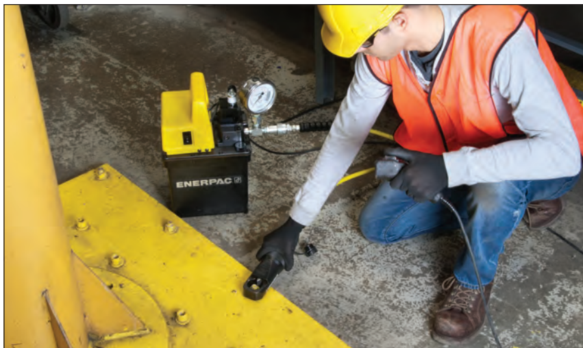
◀ This PED-1101B Submerged pump quickly and quietly powers Enerpac's hydraulic Nut Cutter in this maintenance application.
