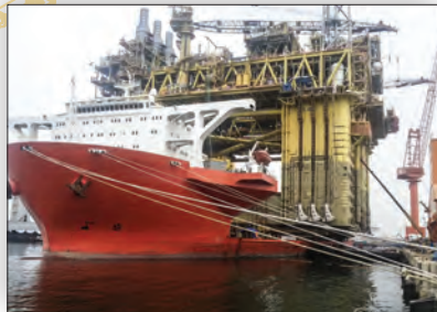
Synchronous superlift and launch
