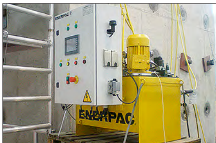
◀ Custom pumps with control packages.
